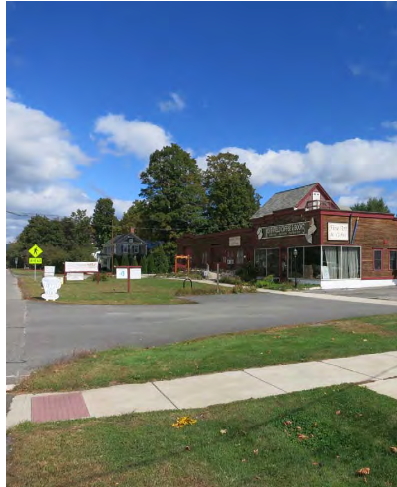
With well-thought-out amendments to the existing bylaw, Northfield could improve the visual character of its streetscape, including the design and placement of commercial signs.
