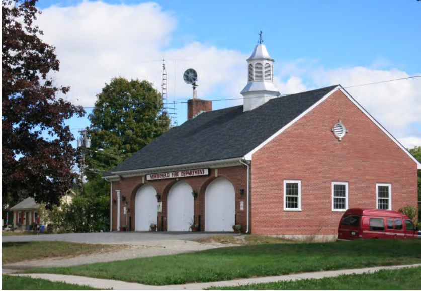
The existing Northfield Fire Department is space-constrained.
