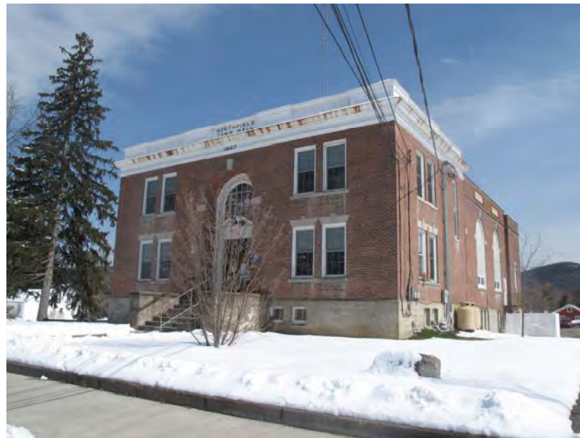
The Town Hall building is in need of repair and renovation.
