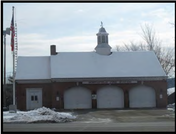
The Fire Station does not adequately store needed equipment.
